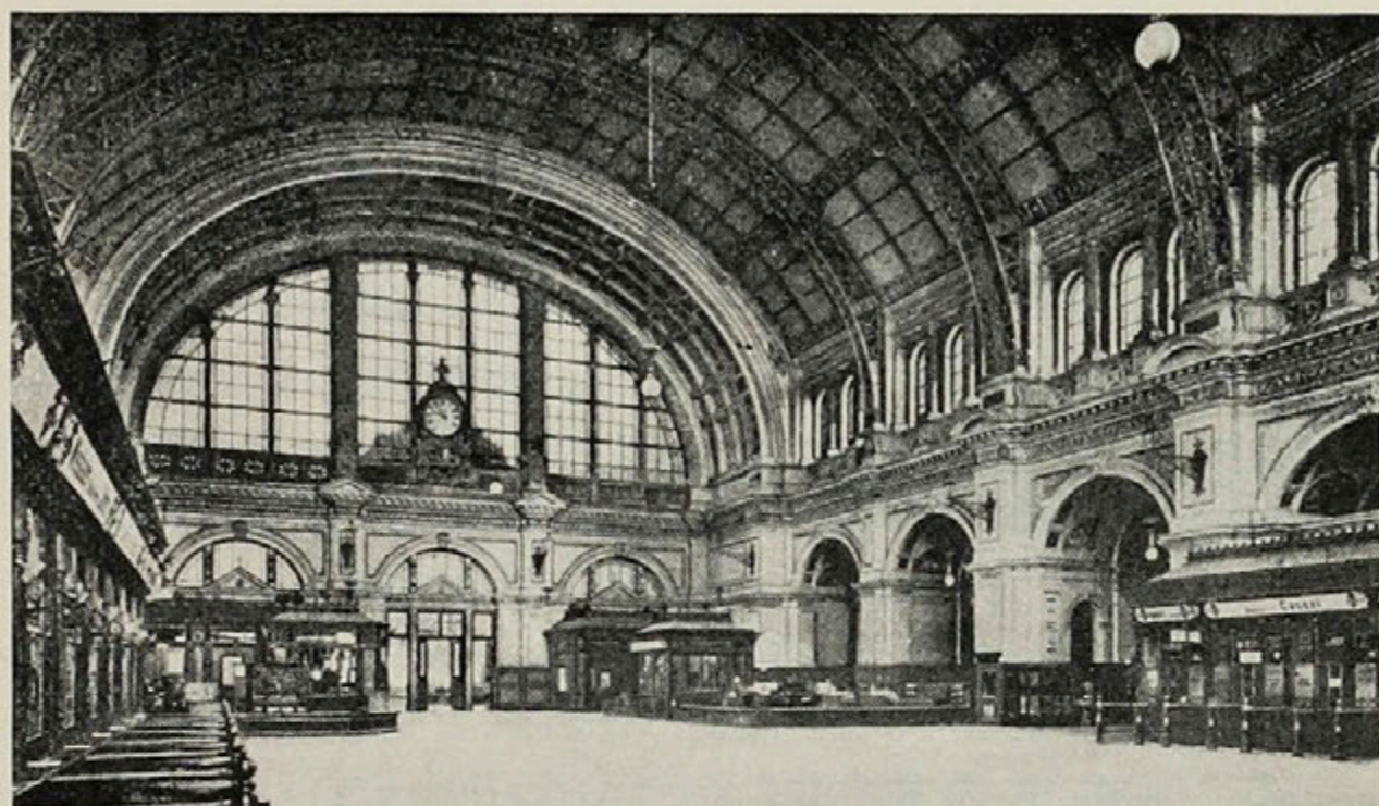
Railway Station, Frankfort-on-the-Main, Germany.
